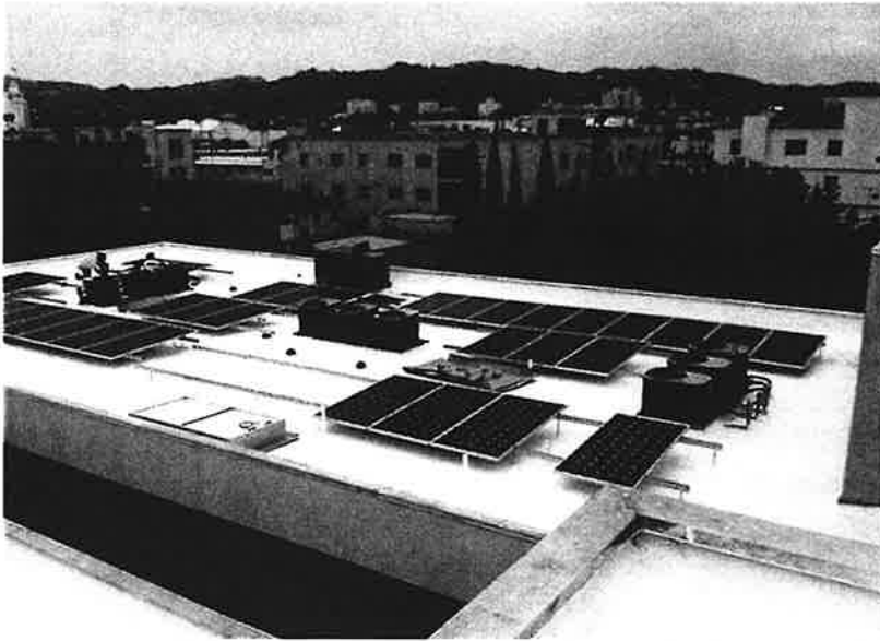
Business installation, flat roof; photo courtesy of Adco. Roofing, www.adco.com
